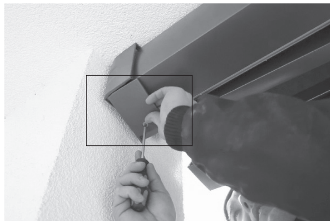
Fig. 12: Mounting covers with awning slightly open
