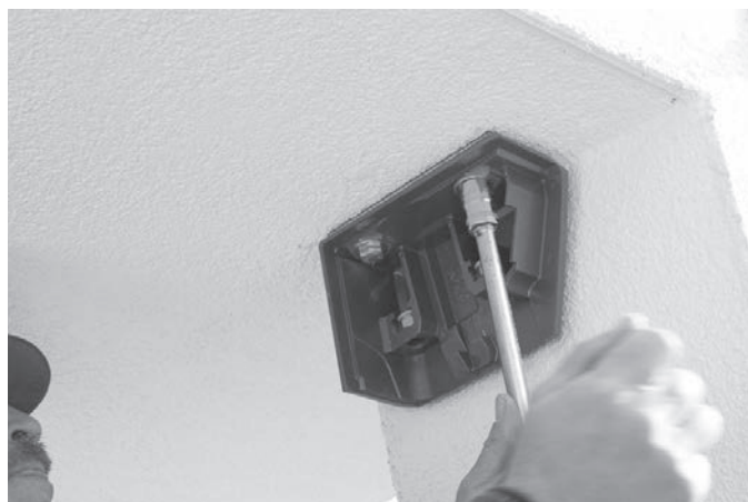
Fig. 08: Tightening fixing screws (ceiling installation here, for example)
