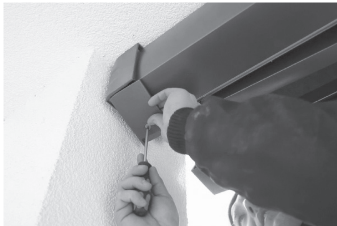
Fig. 16: Remove bracket covers
