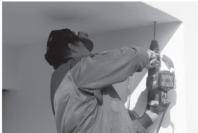
Fig. 06: Drilling holes (ceiling installation here, for example)
